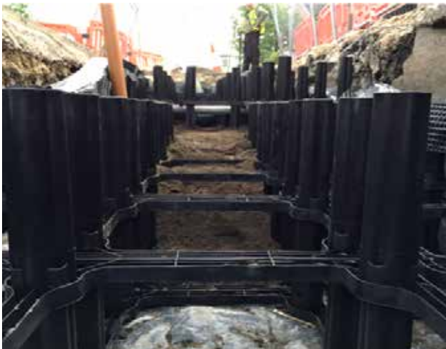
'Box-crate' Tree-planting as a Storage, Water-cycling and Attenuation SuDS Component (images courtesy: DeepRoot UK)
